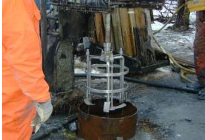
Sampler is lowered into borehole
